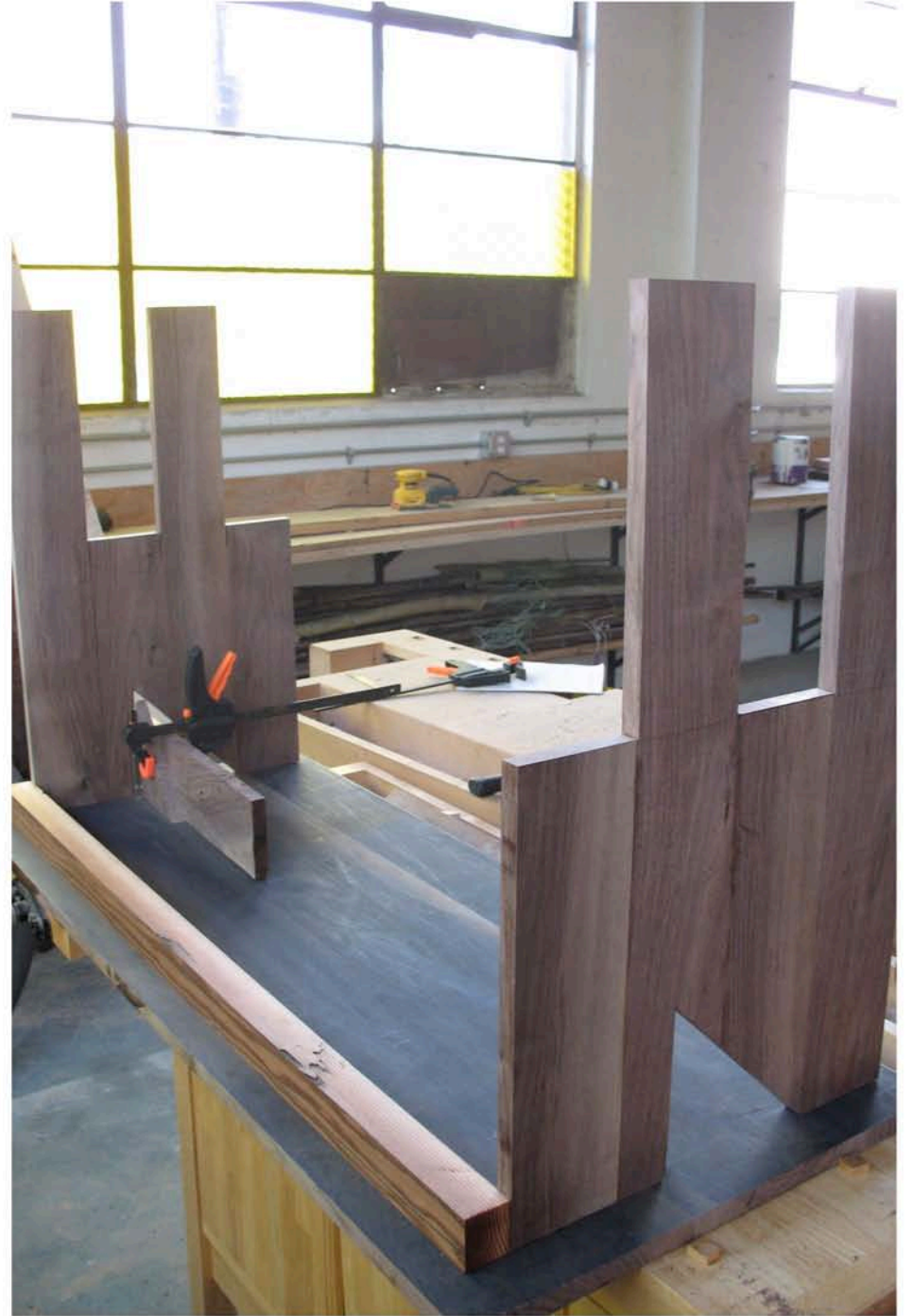
Construction process: Interlocking hinged legs .
